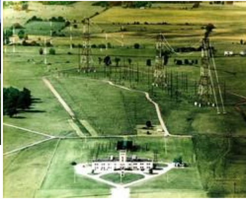
Siege guns: VOA-Bethany's six transmitters were connected to dozens of large antennas spread across a 1-square-mile area. Many people may recall seeing these towers as they drove past on Interstate 75.
